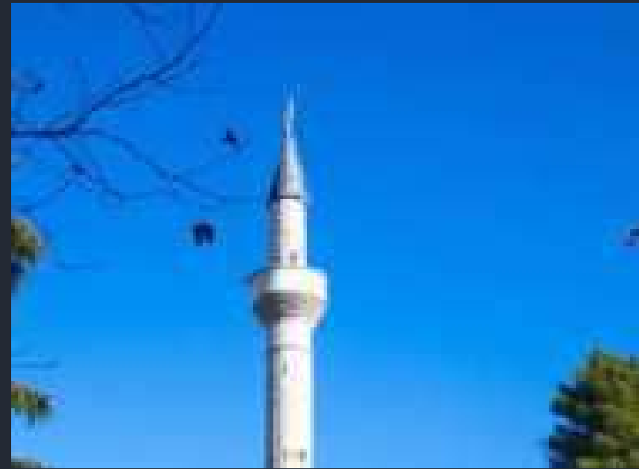
The detail from the Mosque
